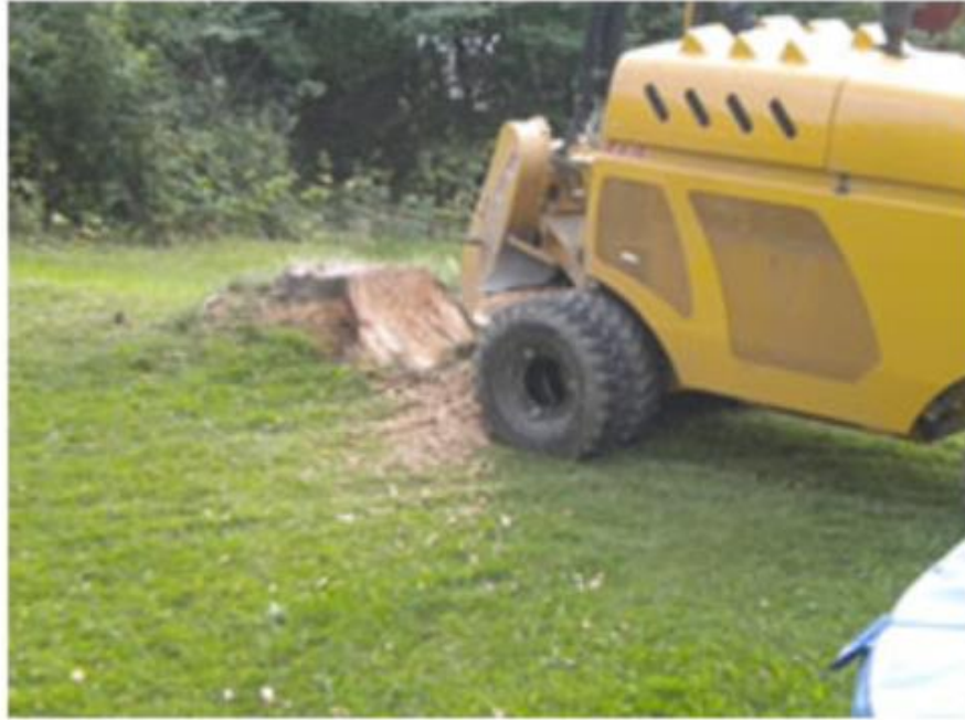
Figure 4: The stump grubber removing the tree stump was a large and noisy machine (left) leaving a large pile of wood chippings (right).
