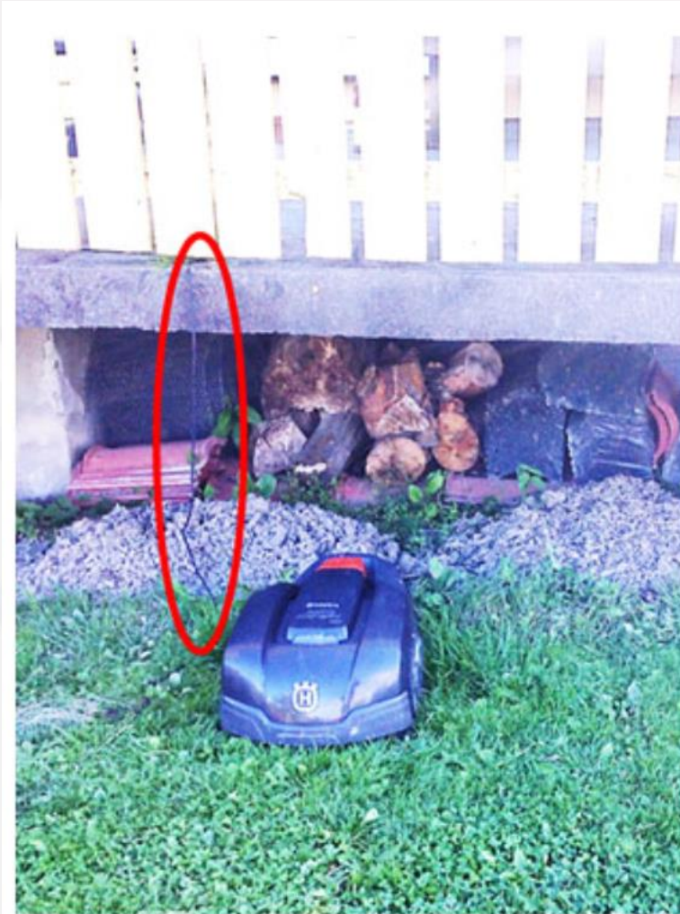
Figure 3: The charging station needed electrical connection and was installed under the veranda. The red line indicates where we first laid the electric cable.
